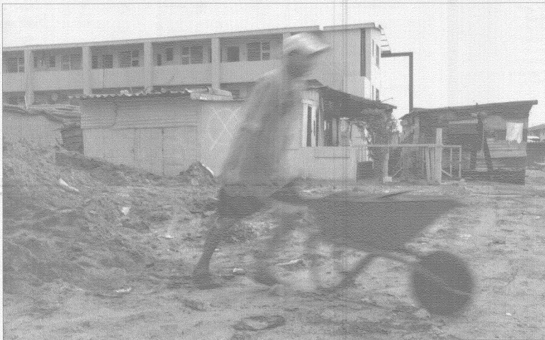
BREAKTHROUGH: So far, the Amakhaya Ngokuk project has provided 232 two-room flats with solar-heated water to the Masiophumelele fire victims of 2006, and a community hall. PICTURE: MICHAEL WALKER
